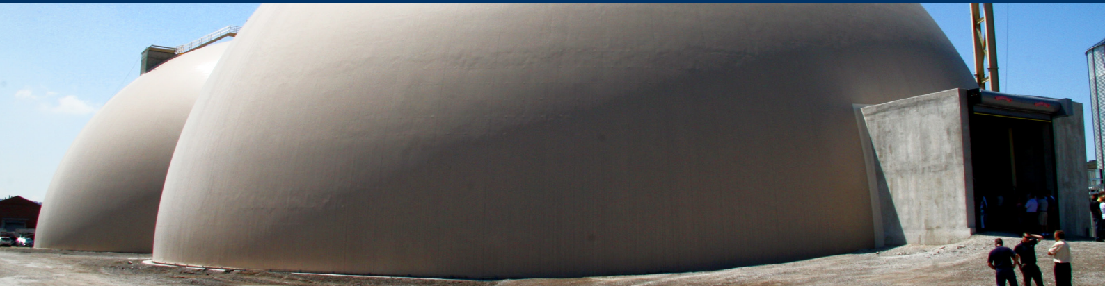
Designed to store grains, sugar, salt or granular fertilizer, these domes have capacity of up to 60,000 tonnes.
