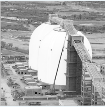
China Coal Hulusu Mine Ordos City, Inner Mongolia, China
