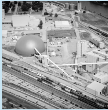
ADM Clinton Cogeneration Clinton, Iowa, USA
