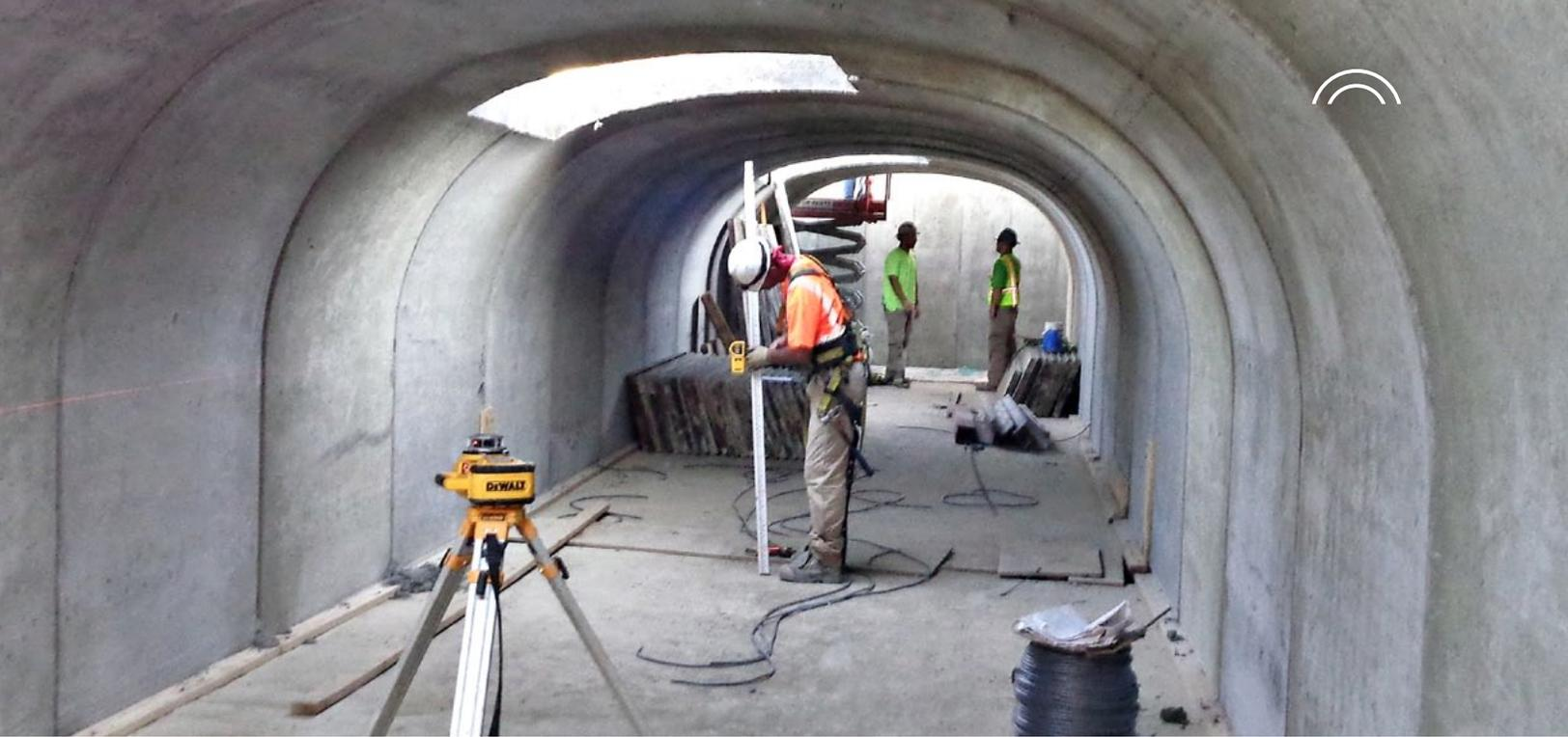
ward with this model. But thousands of tons of product will cause flexural stresses to a flat roof topping the tunnel. To satisfy this flexural demand, the requirement is thicker slabs, more reinforcing, and increased costs.
