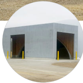
Each salt dome features three truck bays for easing loading.
