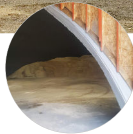
Salt is stacked against the dome wall, freeing up interior space for front-end loader.
