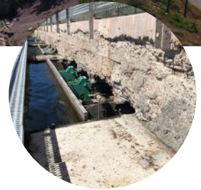
Deteriorating concrete was removed, then replaced with new concrete using the shotcrete method.
