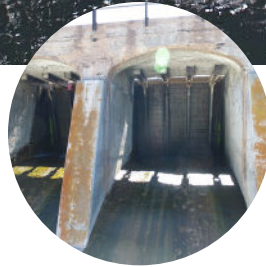
The repaired bays utilize stanchions and flashboards to control flow.
