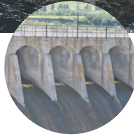
The dam was built in the early 1900s, and the rehab was completed in just over two months.
