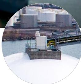
As a result of its geometry, a dome can support sizable structures like a headhouse and conveyors at the apex.
