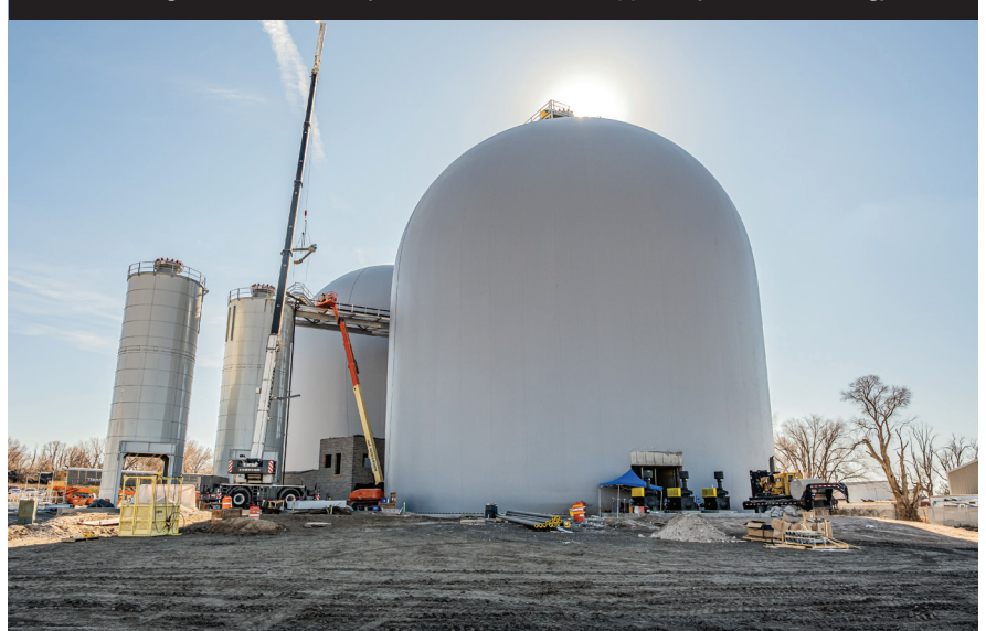
US-based Bridgesource will store fly ash in its new domes supplied by Dome Technology
